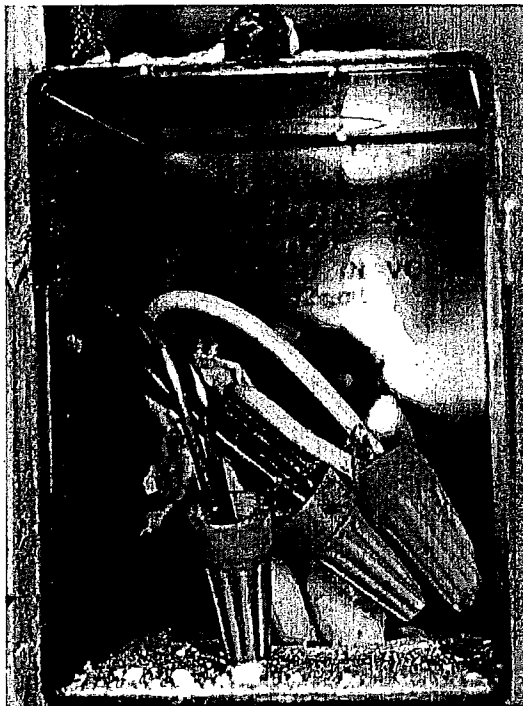
Figure 13. Wire nuts in junction box.
