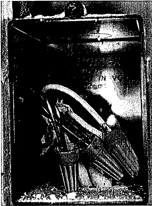
Figure 13. Wire nuts in junction box.
